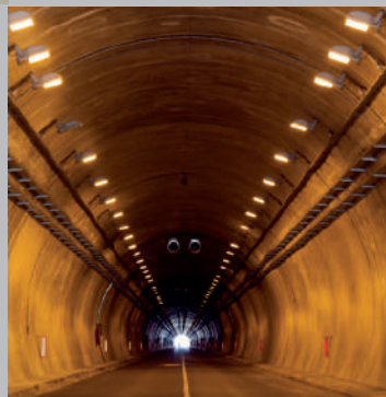
Tunnels and traffic stations
